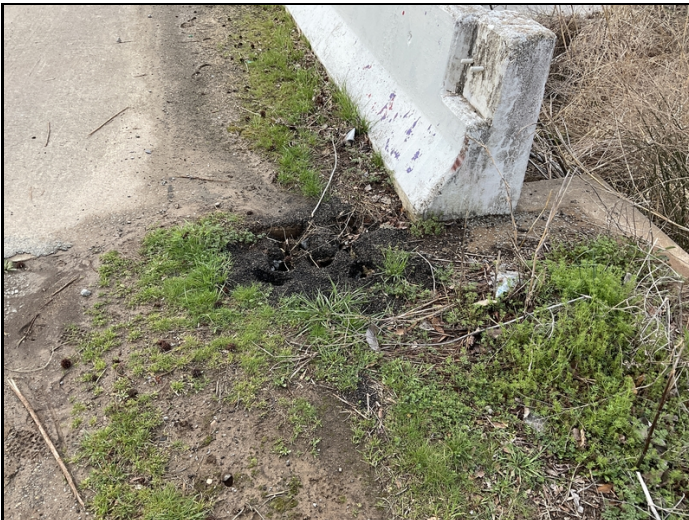
Approach roadway - Bent 4 left: Erosion
