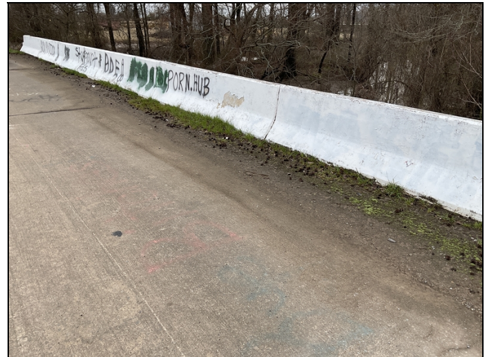
Gutter-line - right side: Debris build-up
