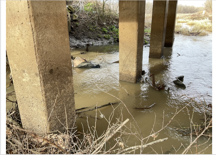
Piling - Bent 2: Abrasive wear
